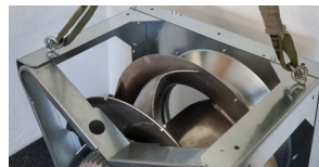
Fitting lifting lugs in the positions provided
